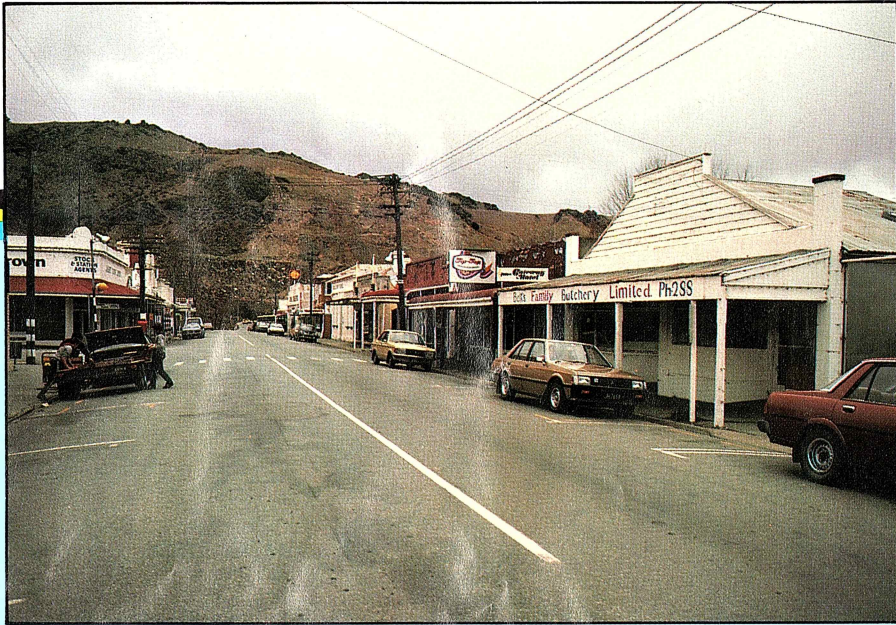
ABOVE: The old commercial area of Cromwell which was demolished in preparation for the filling of Lake Dunstan.
